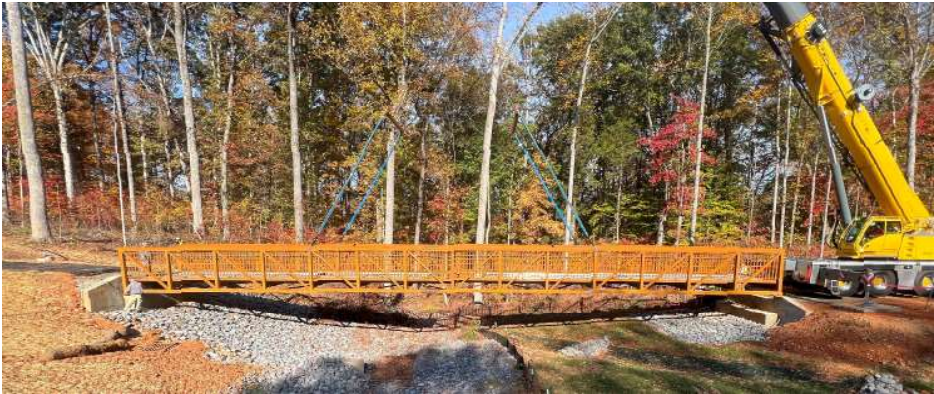
▼ IMAGE 1.4 PHASE ONE BLUE HERON TRAIL PEDESTRIAN BRIDGE INSTALLATION
