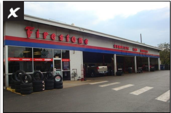
Service bays on primary building wall
