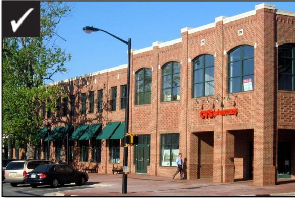
Adequate window area
