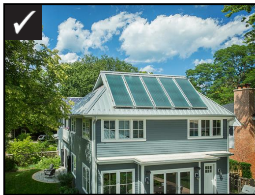
Non-contrasting solar panels on rear of structure
