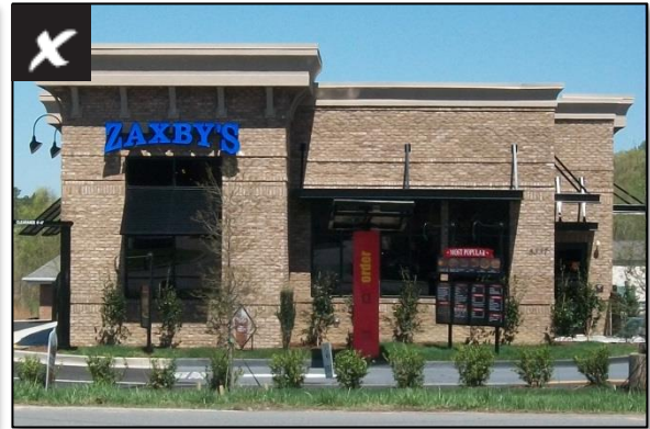
Drive-through ordering station on front facade
