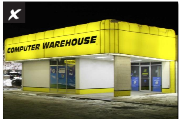
Backlit vinyl awning covering length of building
