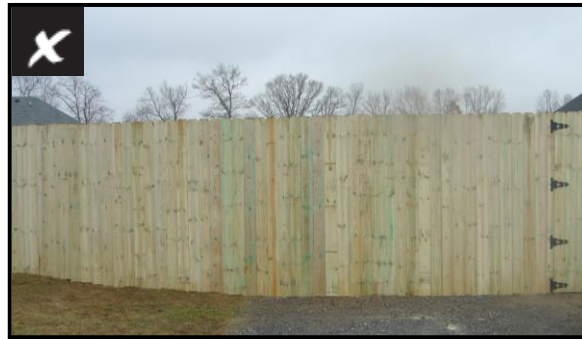
Fence with no Visual Breaks
