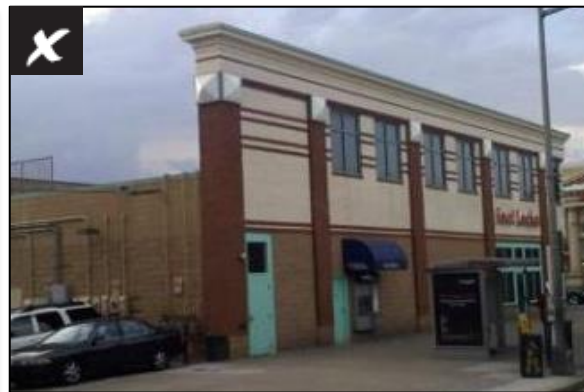
Non-continuous false front parapet
