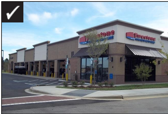
Service bays on secondary building wall
