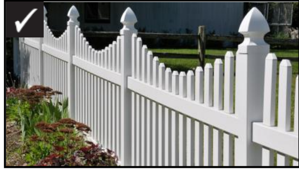
Vinyl Fence and Columns with Decorative Caps
