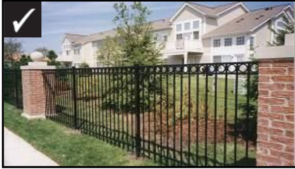
Aluminum Fence and Brick Columns with Decorative Caps
