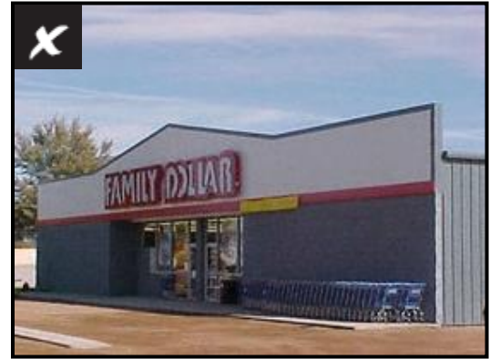
Standard Concrete Block and Metal Facades
