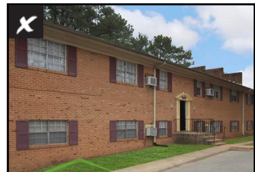
No Wall and Roof Articulation
